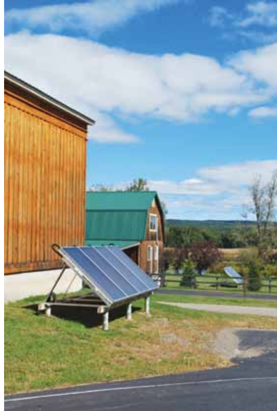
More than 70% of Tierra’s electricity comes from solar panels placed throughout the property.
